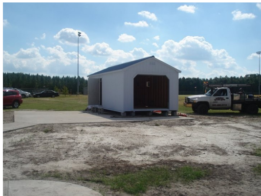
New storage shed
